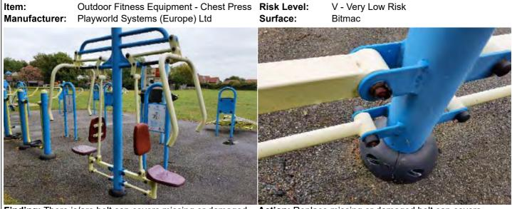
**Finding:** There is/are bolt cap covers missing or damaged on the item
