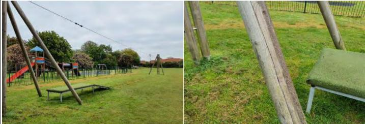
**Finding:** The timber has a number of splits/shakes or air **Action:** Monitor to ensure the splits do not cross through cracks and this may affect the stability or allow water ingress fixing points of the structure and/or cause any instability which will accelerate the rotting process
