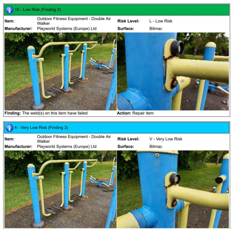
Finding: There is/are bolt cap covers missing or damaged Action: Replace missing or damaged bolt cap covers on the item
