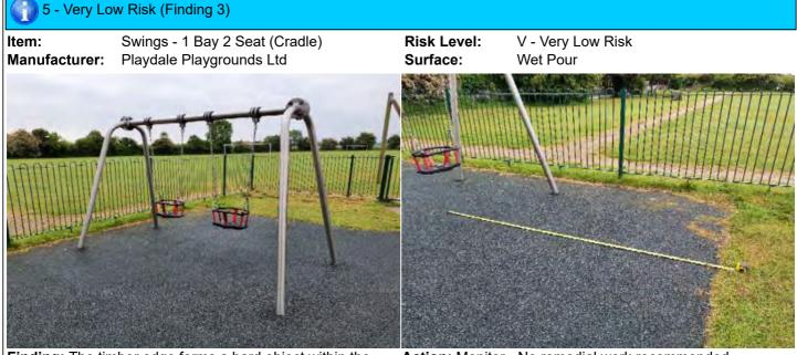
Finding: The timber edge forms a hard object within the impact area of the equipment in contravention of the requirements of BS EN 1176 Part 1
